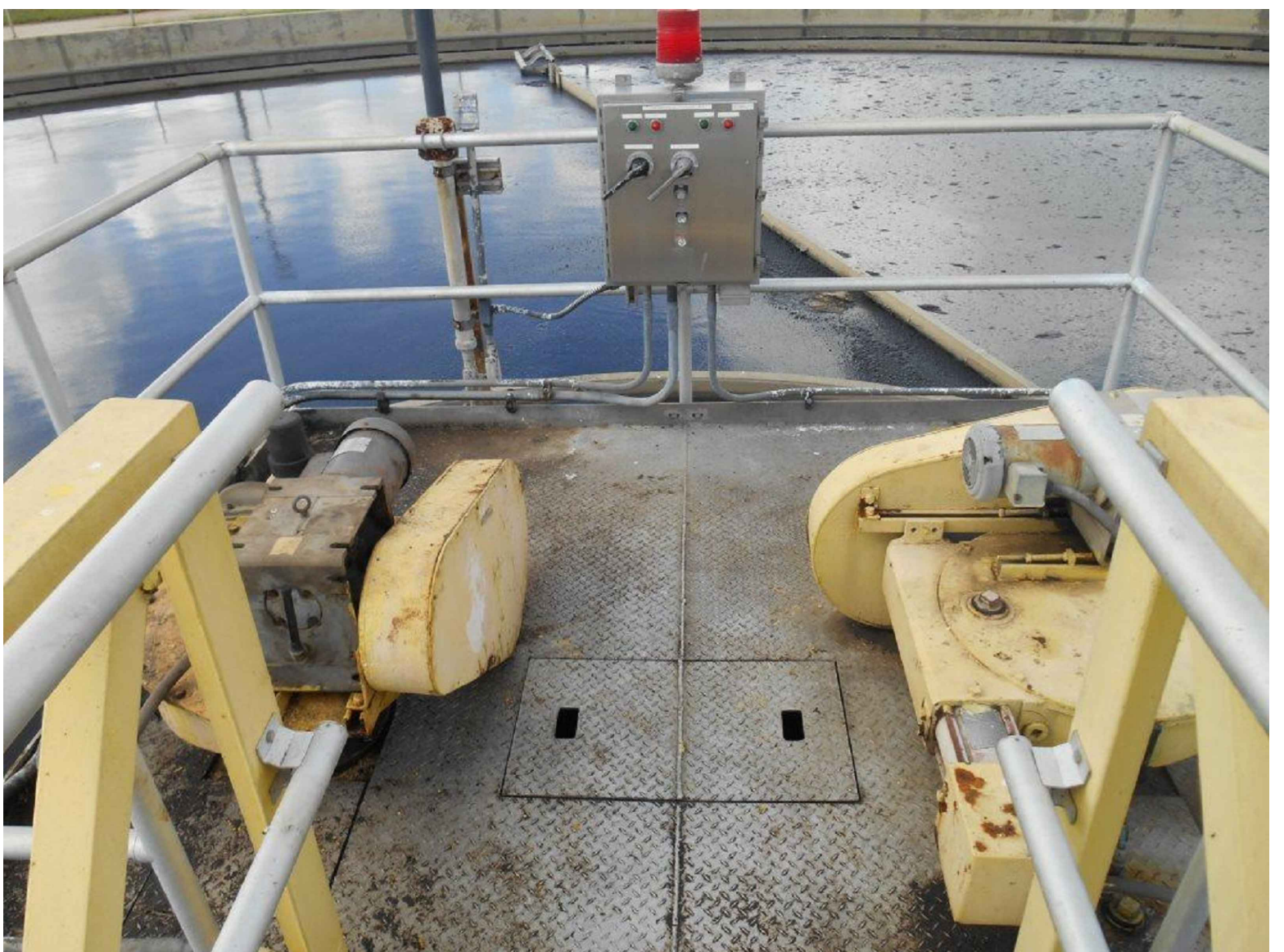
PRIMARY CLARIFIER NO.3 PHOTOGRAPH A
