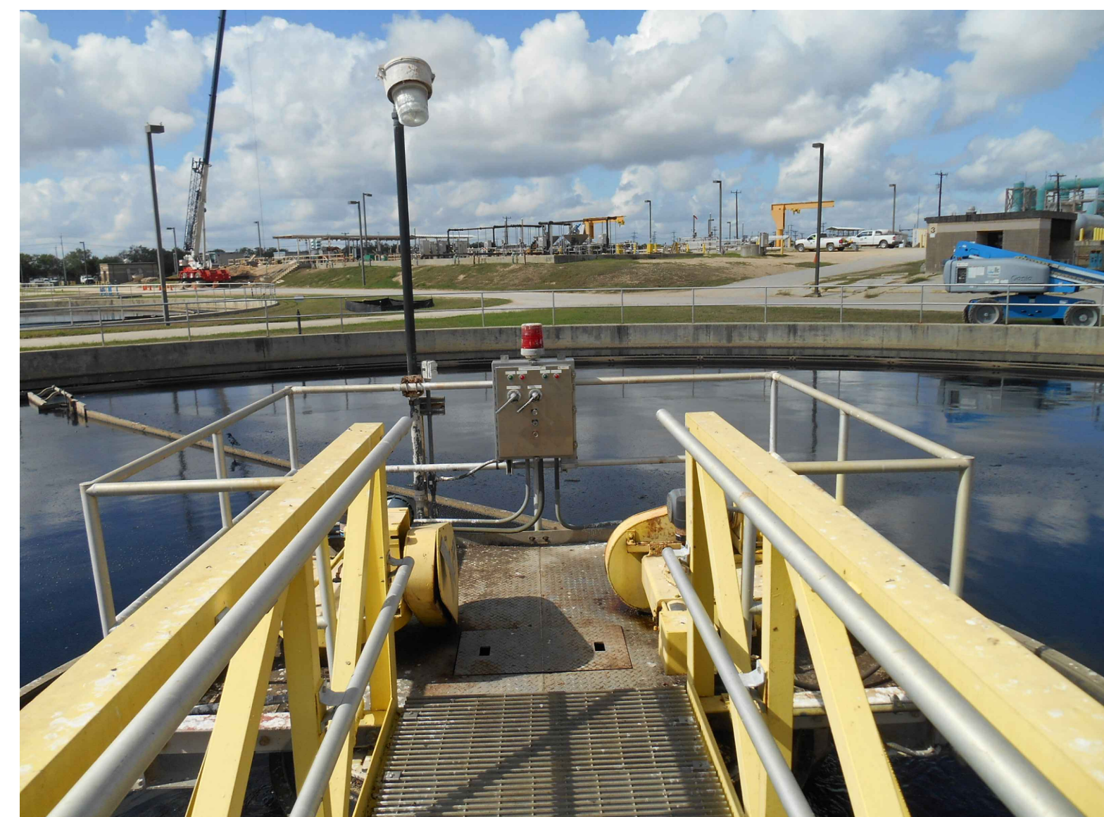
PRIMARY CLARIFIER NO.7 PHOTOGRAPH A
